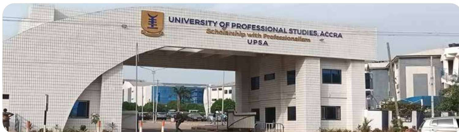
Refurbished Existing Gate House
